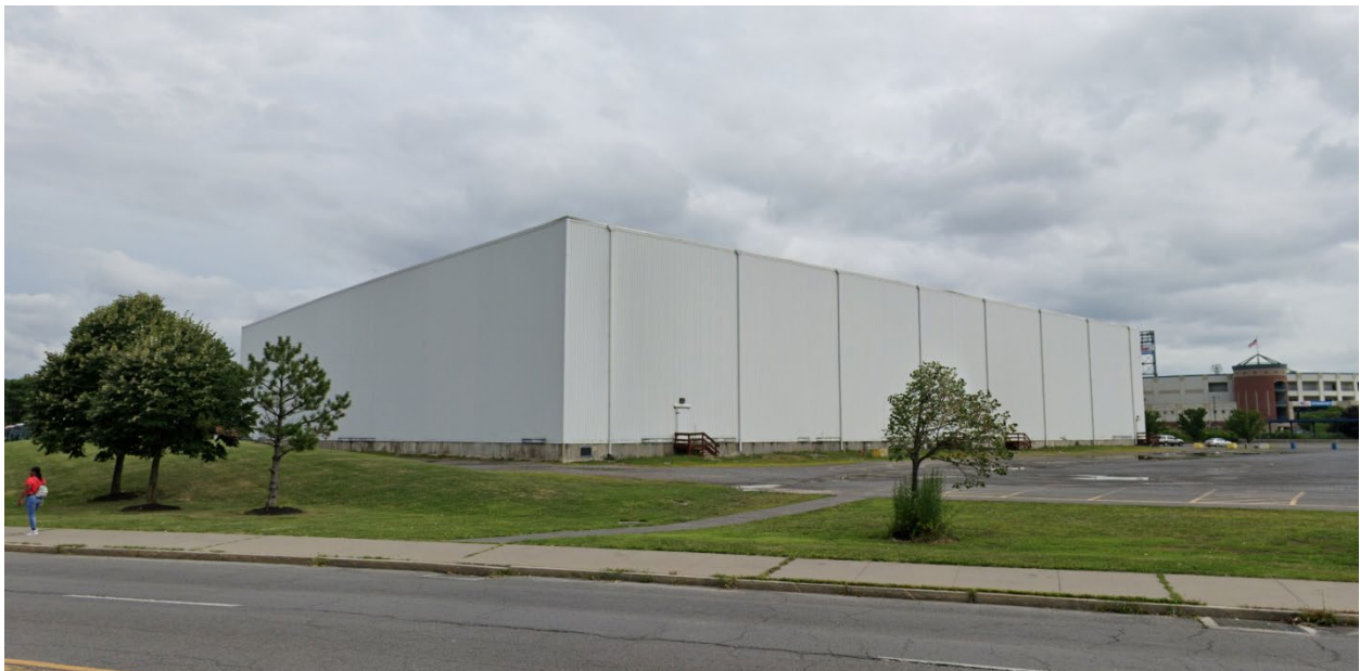
Figure 21. Byrne Dairy Freezer View from NBT Bank Pkwy
