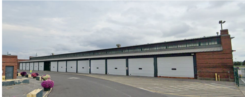
Figure 54. A Shed with Closed Garage Doors
