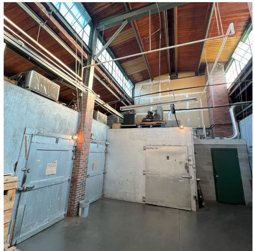
Figure 20. Commission House exterior and interior
