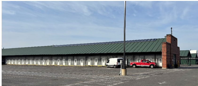
Figure 55. C Shed with Closed Garage Doors
