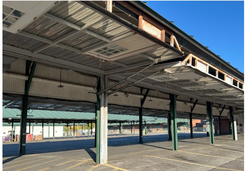
Figure 57. C Shed with Open Garage Doors
