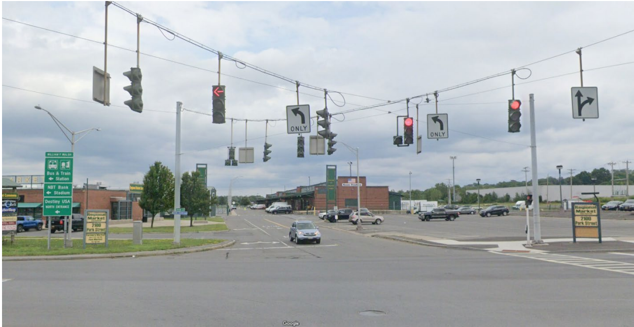
Figure 70. Park Street Entrance
